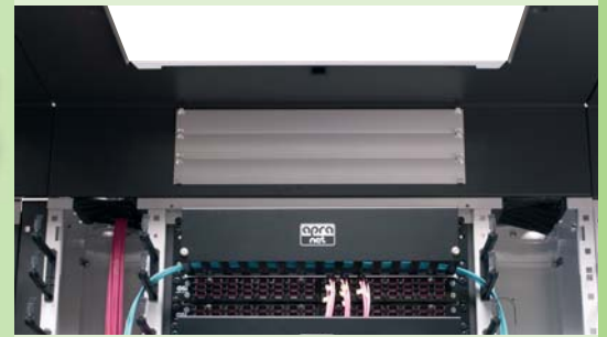
Interior view cool corridor
